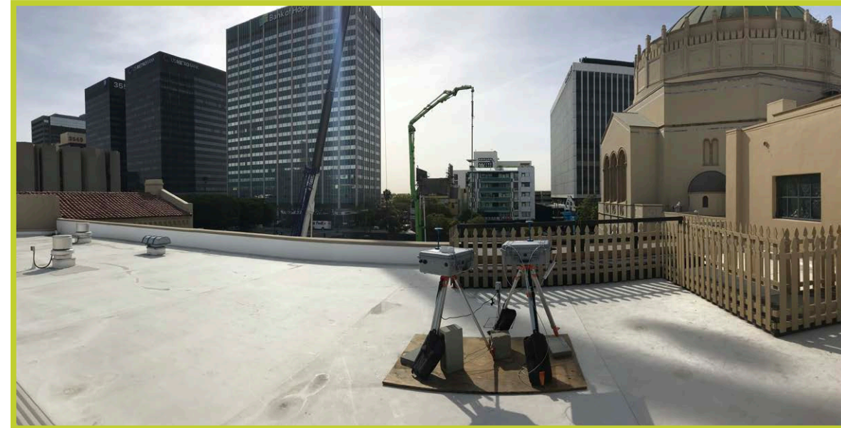
Transit System Construction Project - Los Angeles, CA 2018
