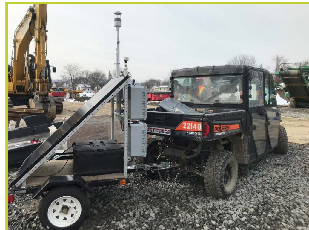
Soil Removal and Remediation Project - Elmira, NY 2022
