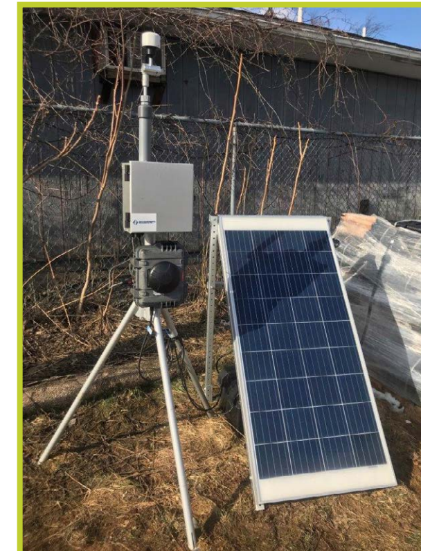
Soil Removal & Remediation Project - Elmira, NY 2022
