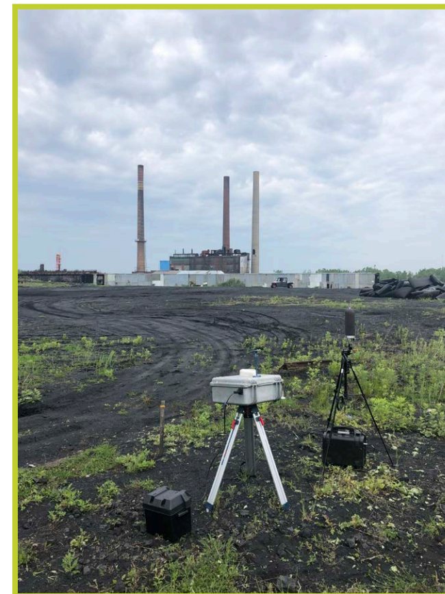
Smokestack Demolition - Tonawanda, NY 2021
